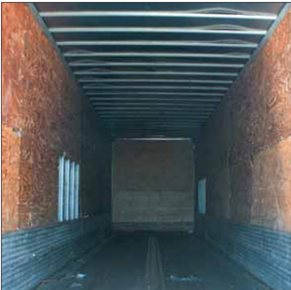
Typical interior damage from daily loading and unloading
